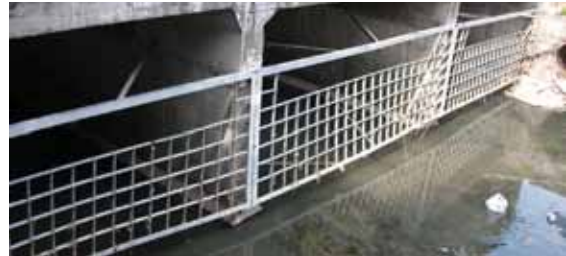
Rubbish traps were installed to ease collection and removal of rubbish as well as to prevent rubbish from flowing to other rivers/tributaries
